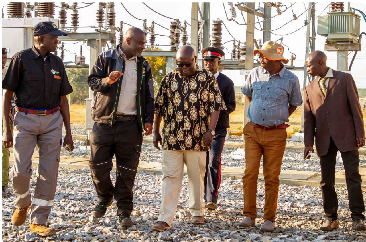
Figure 5: Inspection of the Mitete Grid Extension Project led by the Minister of Western Province, Hon. Kapelwa Mbangweta M.P.
