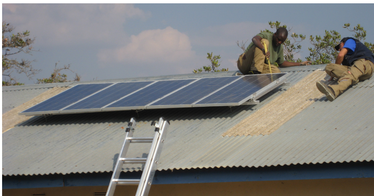
Figure 8: Installation of High Powered Solar Home System at a School
